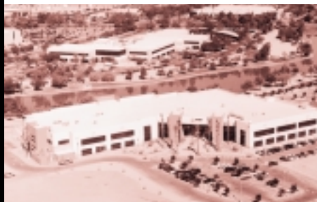
Avnet Computer Marketing's new global headquarters, a 132,000 sq. ft. facility at Arizona State University's Research Park, Tempe, Arizona.
